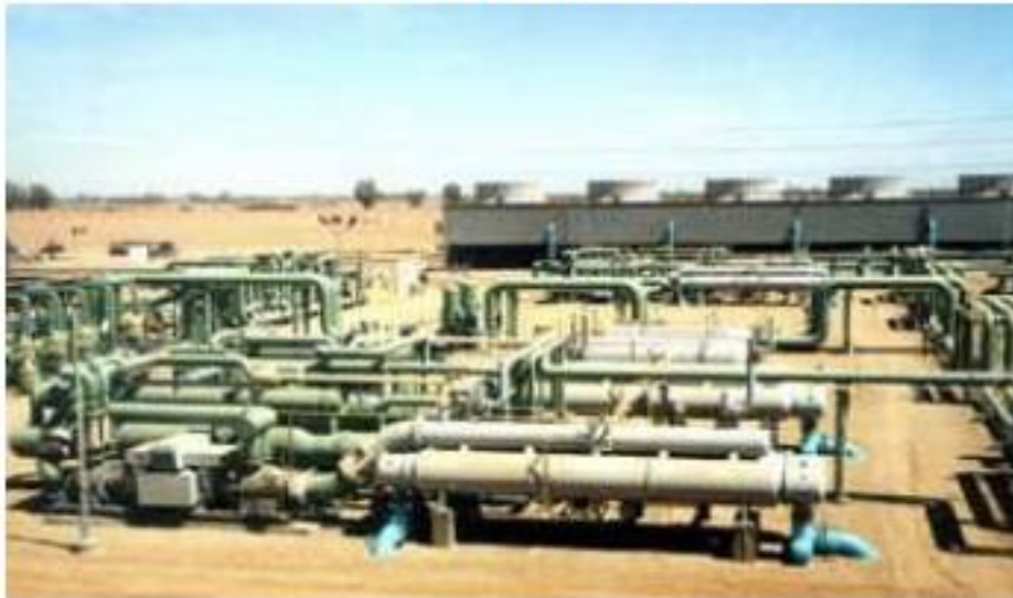
Ormat SIGC Binary Plant (SIGC) with Water Cooled Condensers
