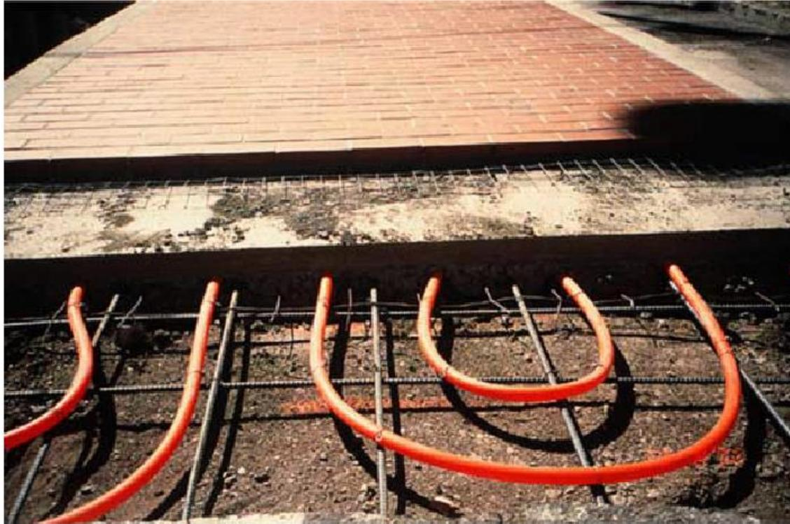
Pipes of geothermal water can be installed under sidewalks and roads to keep them from icing over in winter, like this sidewalk.
